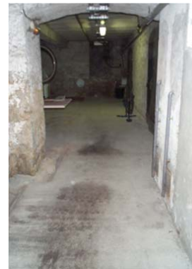
Cellar floor: concrete
