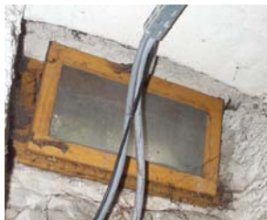
Basement: opened window
