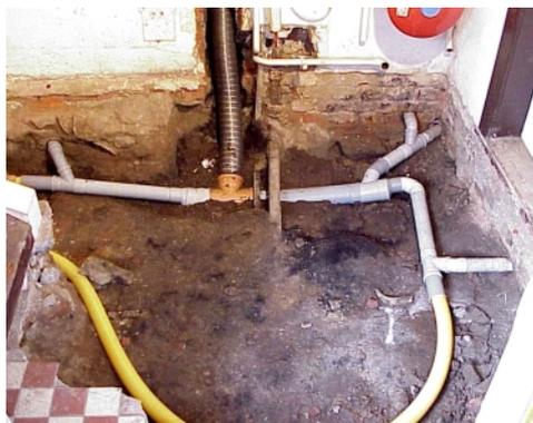
Chase excavated in the entrance hall served for drilling of perforated tubes into the sub-floor layers under the adjacent rooms. Horizontal PVC-U pipe connects the drilled tubes to the vertical exhaust from flexible rustless pipe, which is inserted into a free flue.
