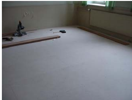
New floor, about 3 cm thick
